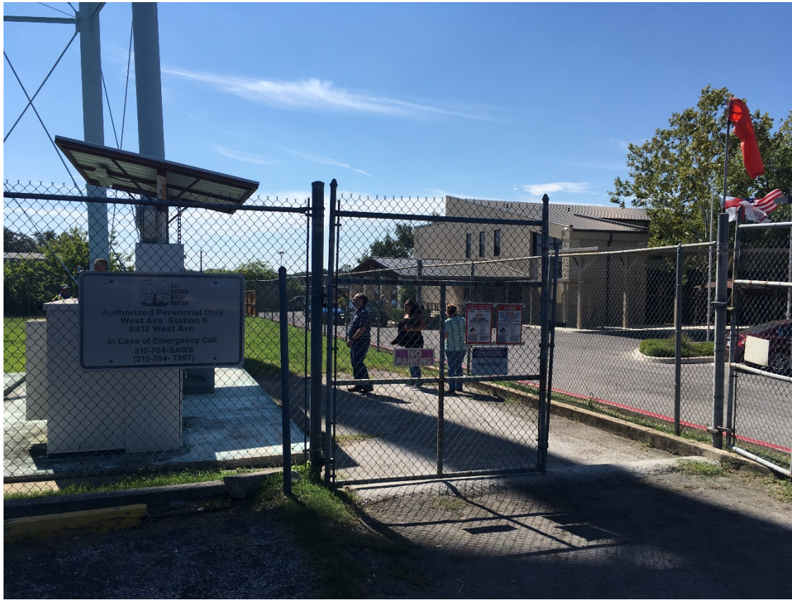
Fence and Gate Replacement
