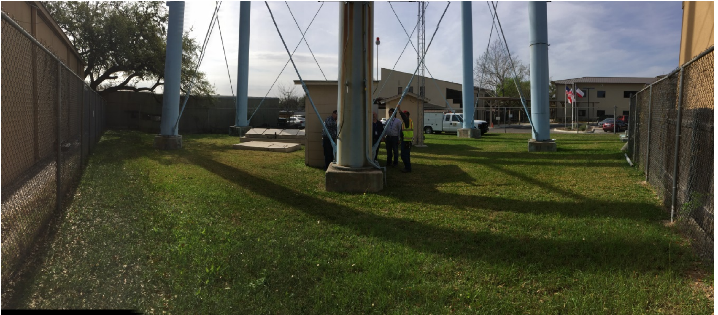
West Avenue Elevated Storage Tank Rehabilitation Painting Project
