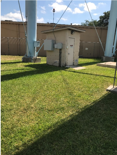
Chlorine Feed Building
