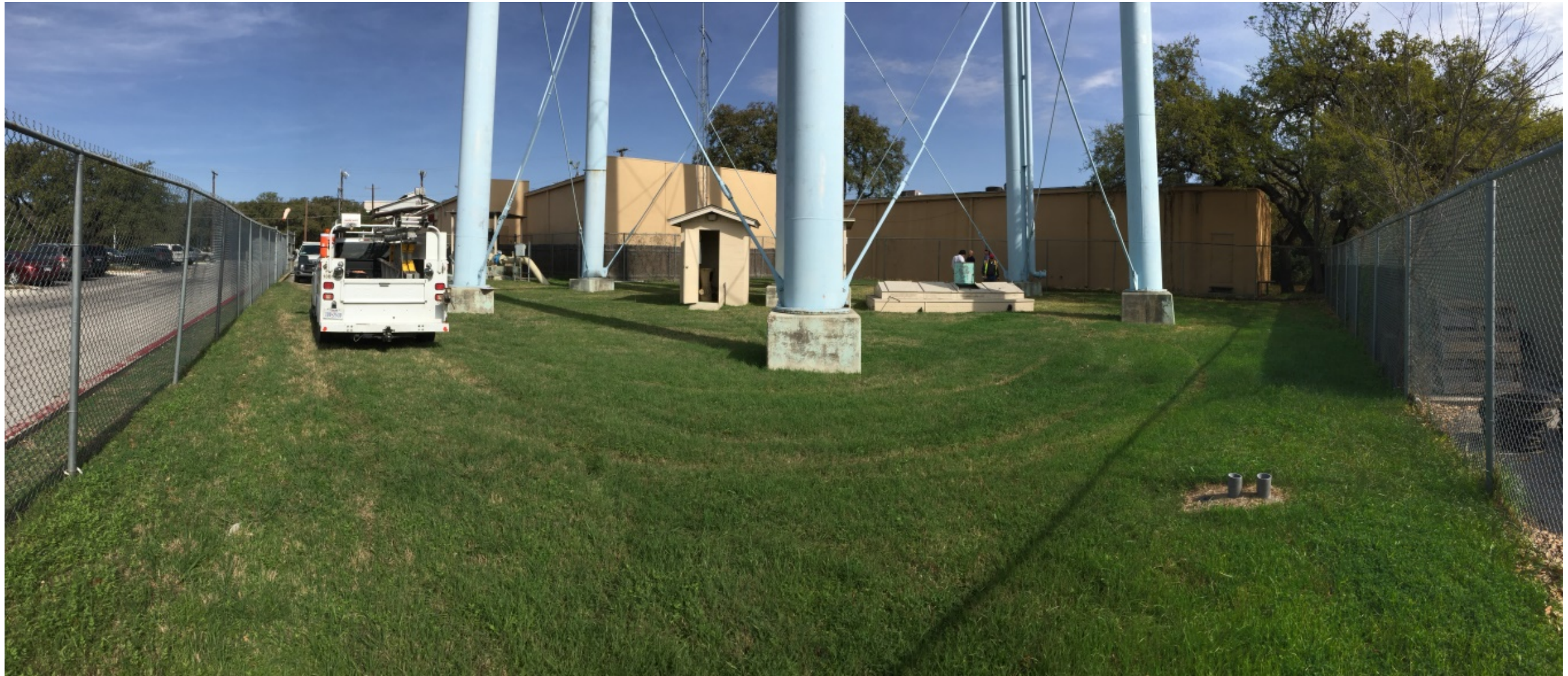
West Avenue Elevated Storage Tank Rehabilitation Painting Project
