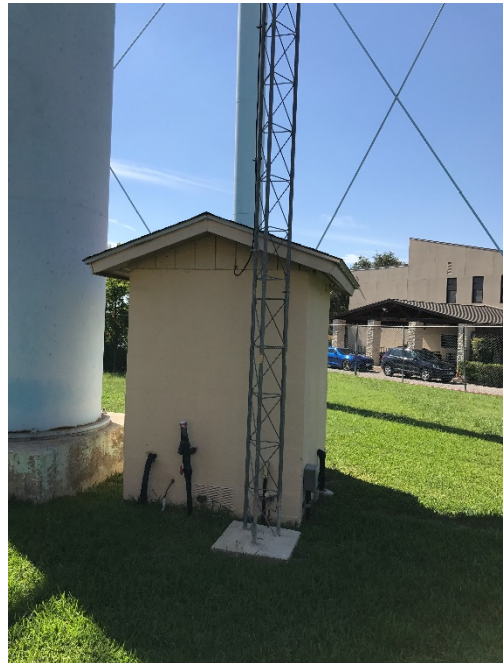
Chlorine Booster Pump Building
